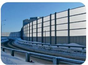
Fibrolite plates are the main filters of noise reduction which are established along the railroads and highways
